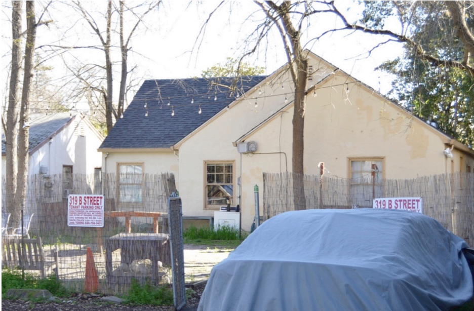
Figure 1. Rear elevation with cross gables, looking east.
